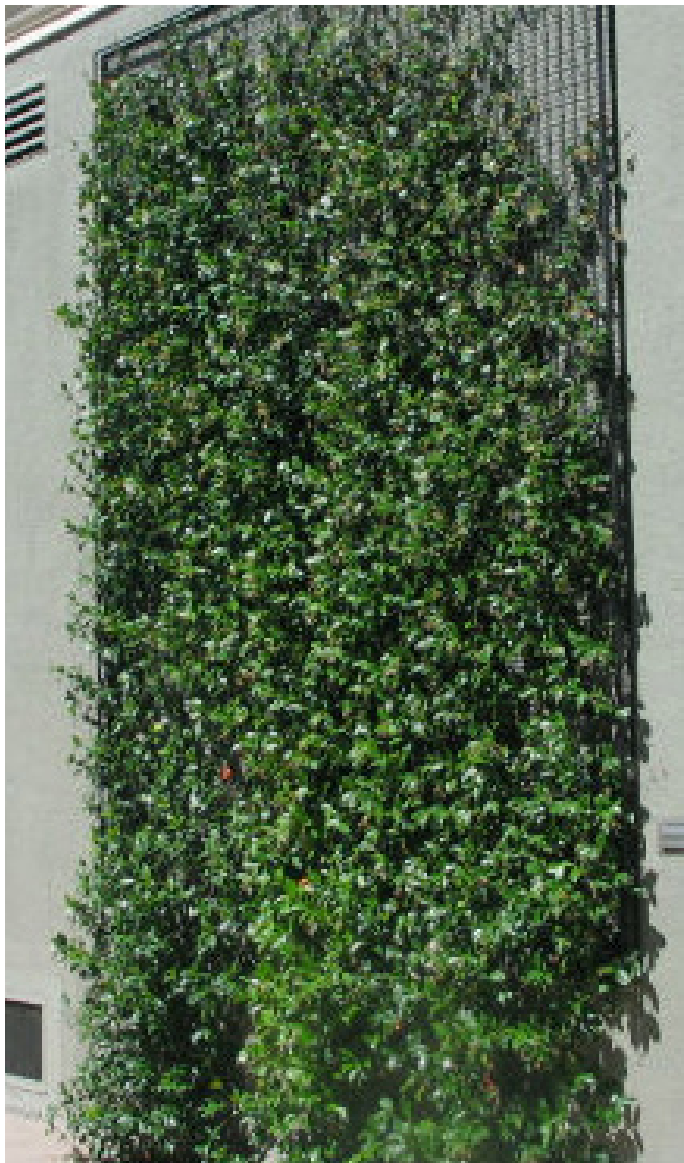
Green facade: Wire mesh & climber from planter
